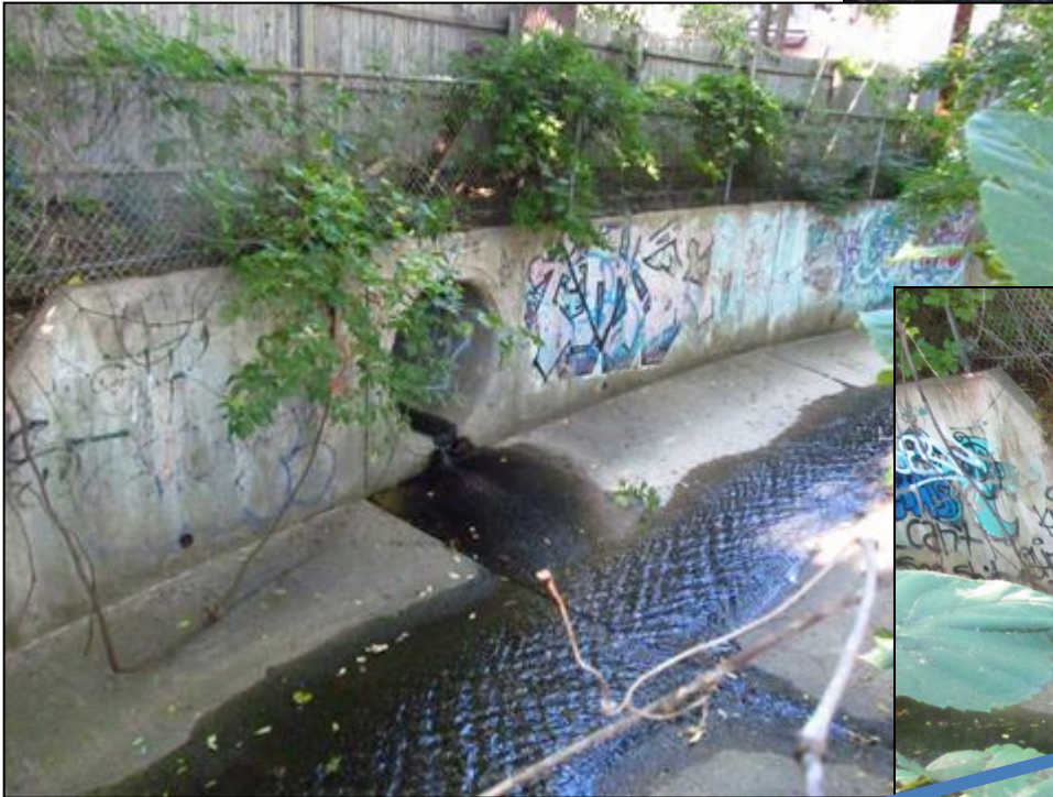
Storm Drain Inlet
