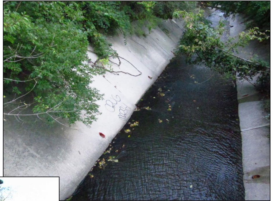
Looking downstream at the Willett Branch from the bridge
