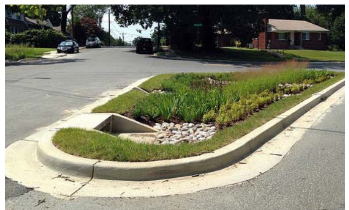
Above left and right: Examples of median treatment for stormwater runoff. From the Dennis Avenue Montgomery County Green Streets project.
