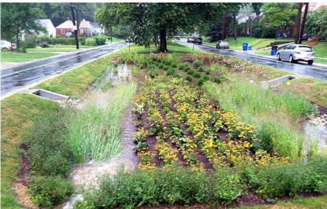
Above left and right: Examples of median treatment for stormwater runoff. From the Dennis Avenue Montgomery County Green Streets project.
