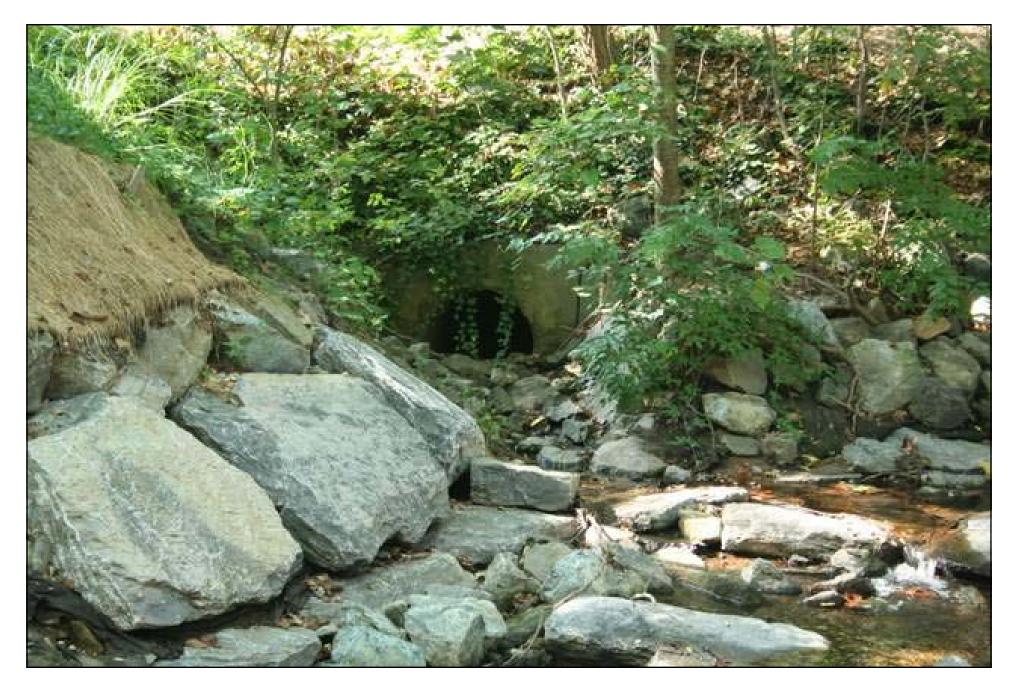
Here we have large rocks and netting to stabilize the stream bank. This replaced the old erosion control method of tarps and riprap. The rocks were first added in 2001. In 2008, another row of rocks was added to the bottom as the creek undercut the first set. You can also see another storm drain inlet. The inlet is being buried and filled in by dirt carried down the storm drain system.
