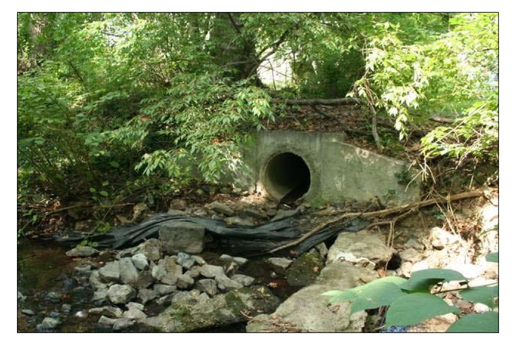
One of the three storm drains inlets from the Town of Somerset. Here you can see remnants of a past erosion control project. The black tarp was laid under rocks to slow the water emerging from the conduit. Unfortunately, the water moved the rocks leaving just the tarp!
