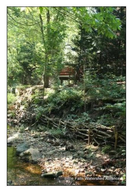
In 2008, bundles of sticks were added to the bank to try to stabilize it to save the property of this house built less than 50 feet from the creek. New regulations discourage building within a stream buffer.
